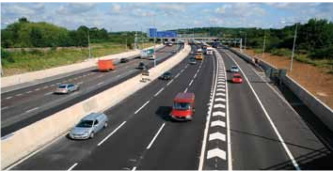
A section of completed motorway and slip road, incorporating most of the slip-formed concrete components used on the M25 project.
