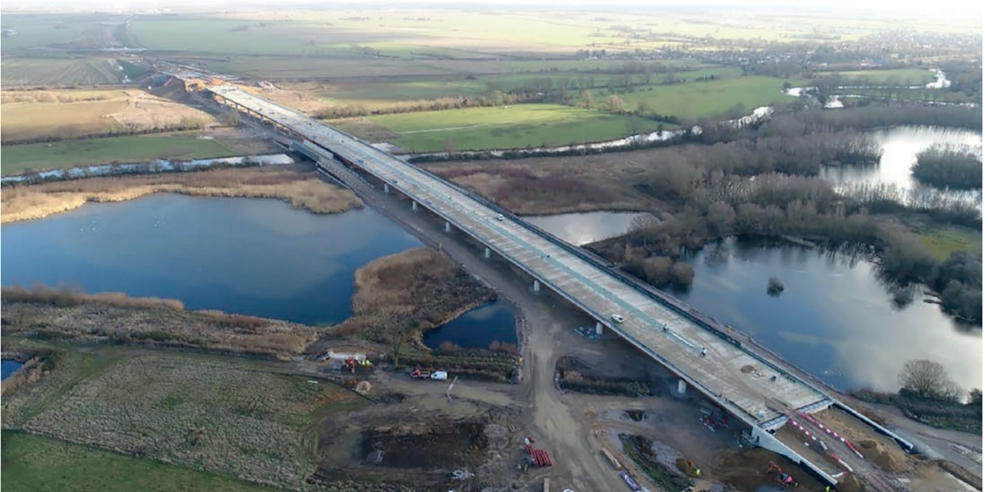
Building work on the new bridge has been completed. Credit: Highways England
