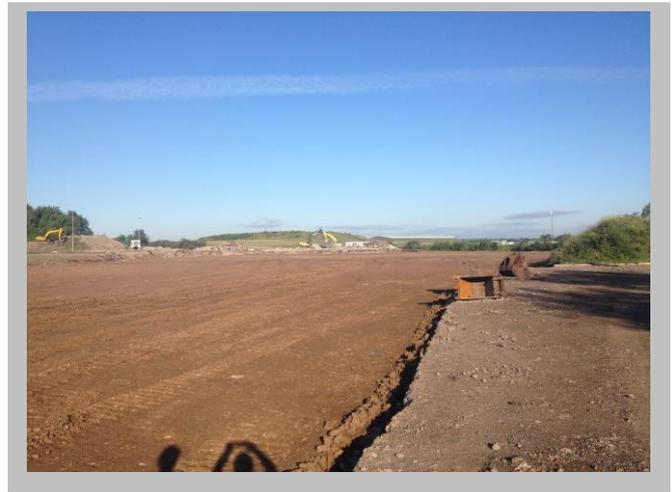
The project involved soil stabilisation contractor C J Pryor Stabilisation improving the soil by importing clay and improving with lime to achieve an engineering fill to enable the building of a new biomass facility.
