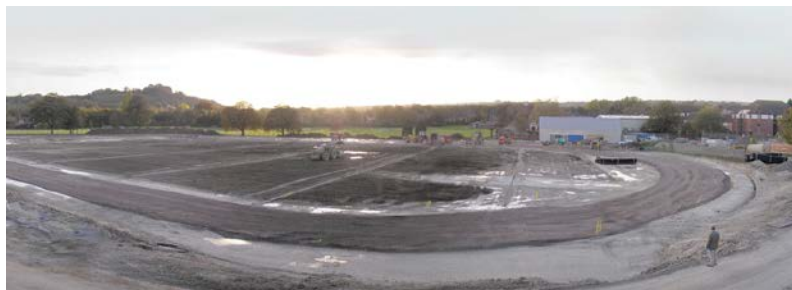
Winchester Athletics Track at stabilisation stage of construction
