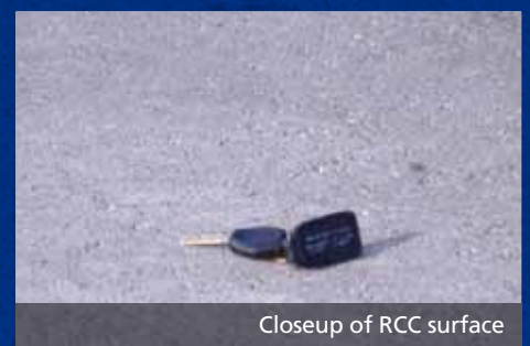
The new hardstanding at Immingham
