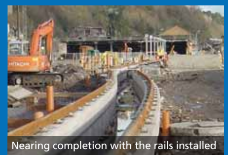
Slipforming the plinth wall at Kent Station
